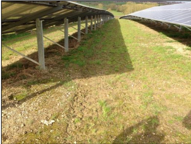
Plate 10.11 Typical thin Racking System driven into ground
