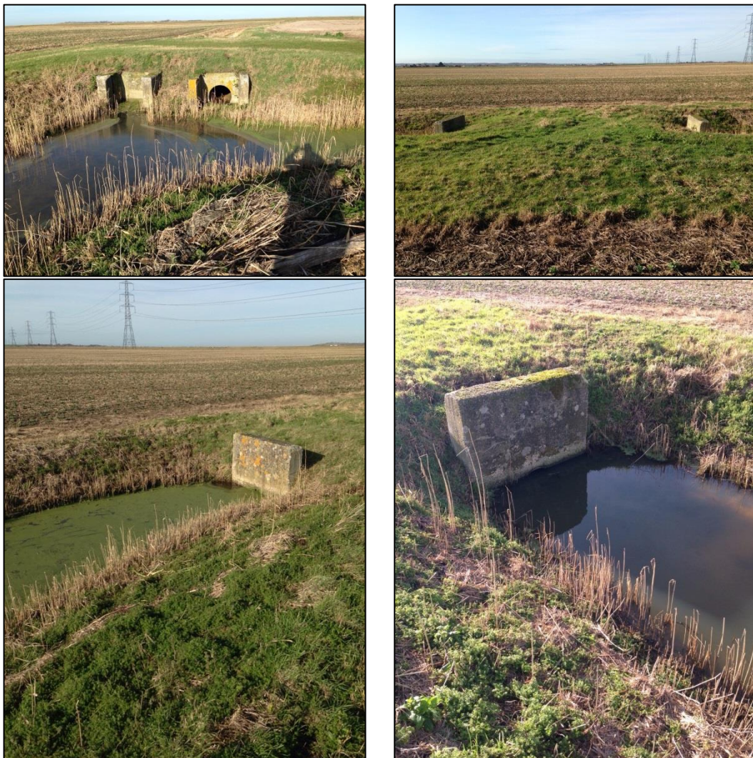
Plate 10.7 Manmade flow control structures within drains
