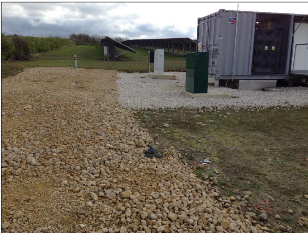
Plate 10.12 Typical Type 2 aggregate at a solar farm 54,55
